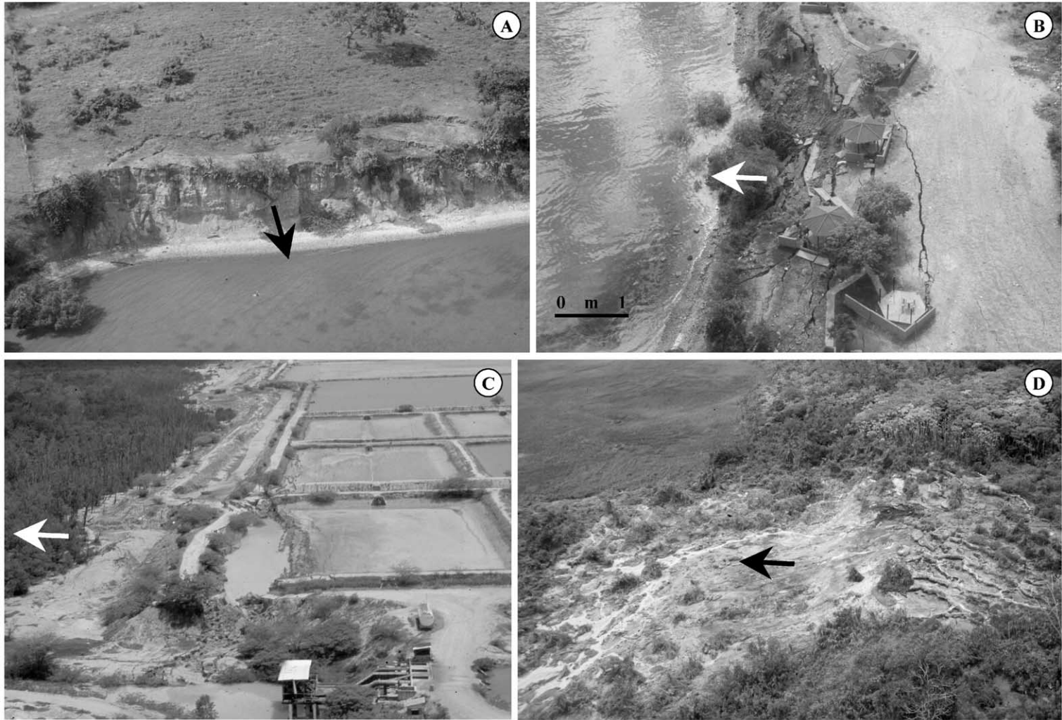
Plate 3. (A) Small lateral spreading in few-meter-high Plio-Pleistocene cliffs on the northern coast of the Cariaco Gulf, nearby Chiguana (for location, refer to Fig. 11); (B) lateral spread affecting small resting area sitting on artificial fill, at the Calzadilla beach, on the southern coast of the Cariaco Gulf; (C) bird's-eye view of seaward lateral spreading of the southernmost earth embankment of the Aquacam C.A. shrimp farm, east of Chiguana; and (D) sliding of travertine pools originally capping the El Pilar fault scarp developed on Mesozoic mudstones at the Aguas Calientes farm. To the south, some unbroken pools can be spotted, whereas travertine blocks are piling up to the north (left). Arrows indicate the direction of sliding.
